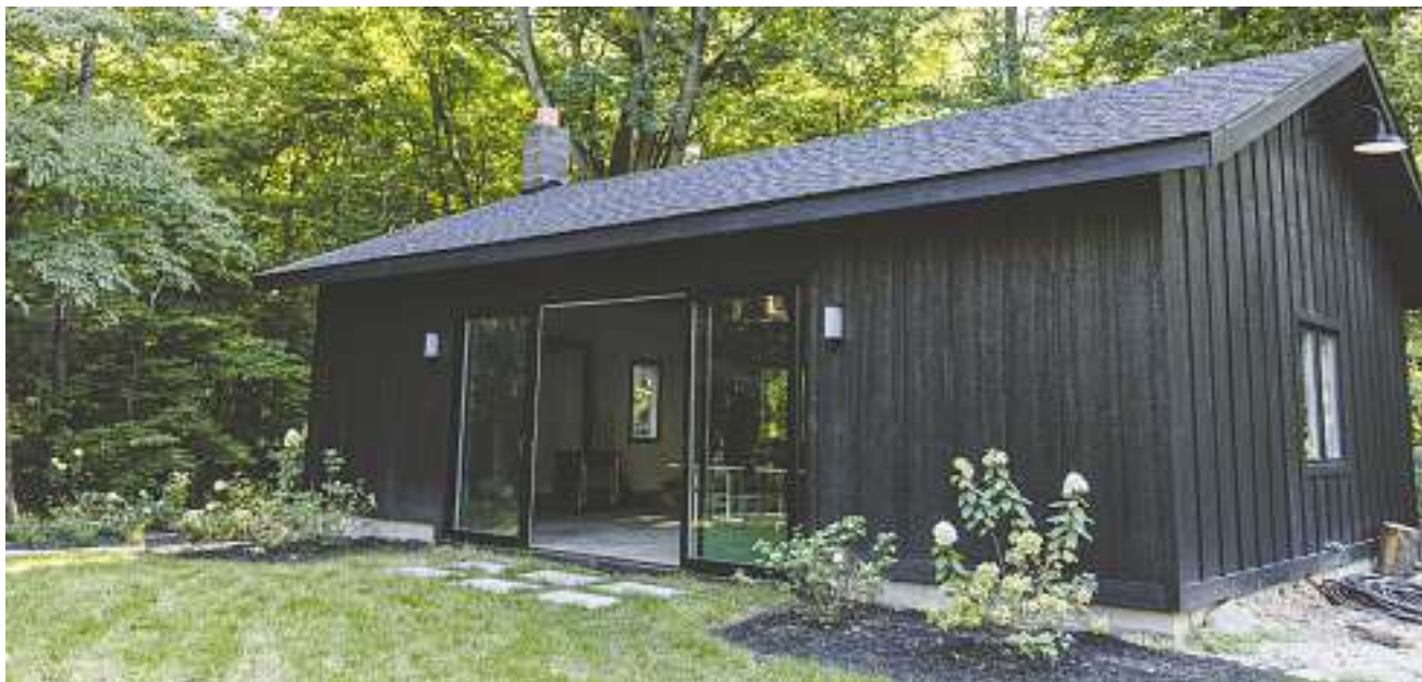
A garage became a detached rec room, also clad in vertical siding painted black.
